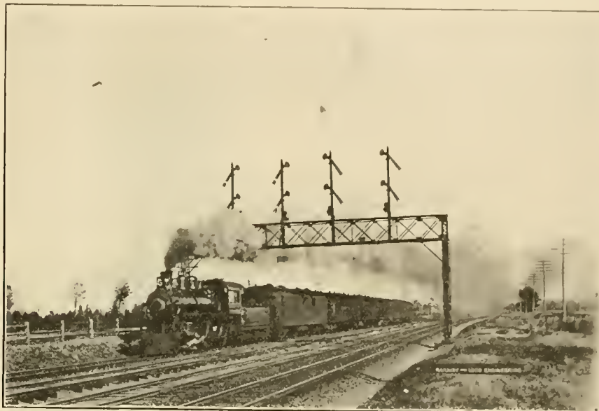
MODERN RAILROAD SIGNAL BRIDGE. LINE CLEAR!
